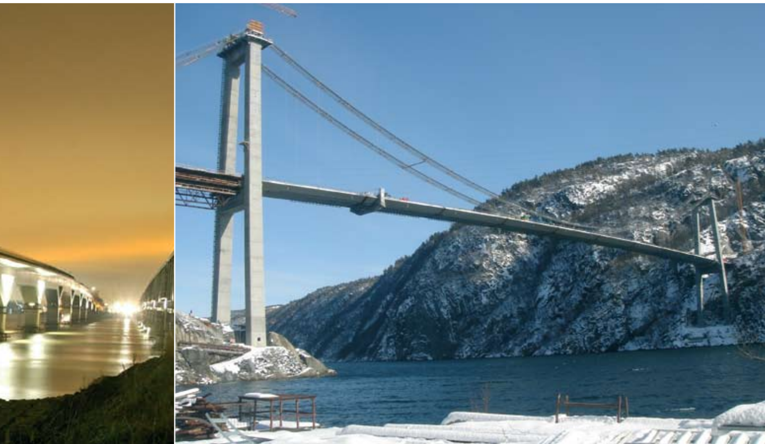
Suspension bridge Fedafjord, Norway
