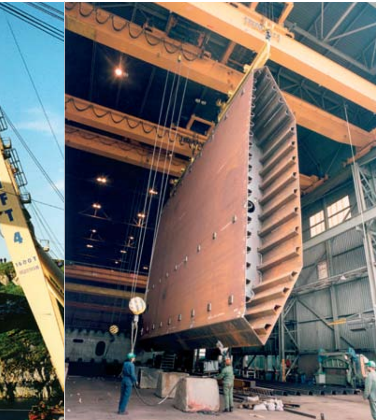
Yard Schiedam, the Netherlands
