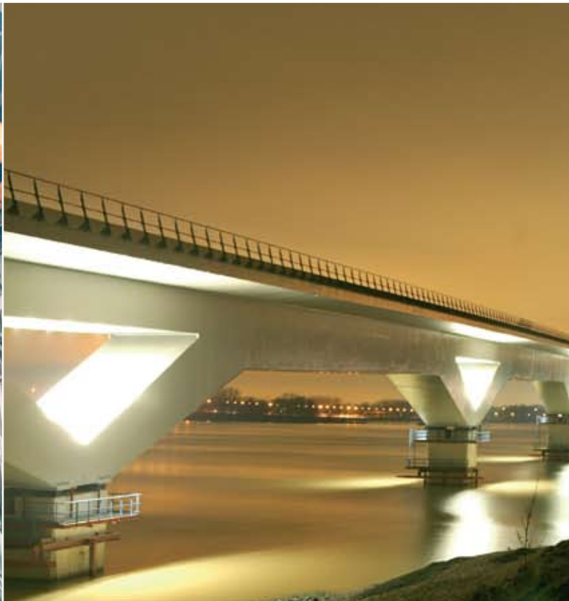
High Speed railway bridge, Moerdijk, the Netherlands
